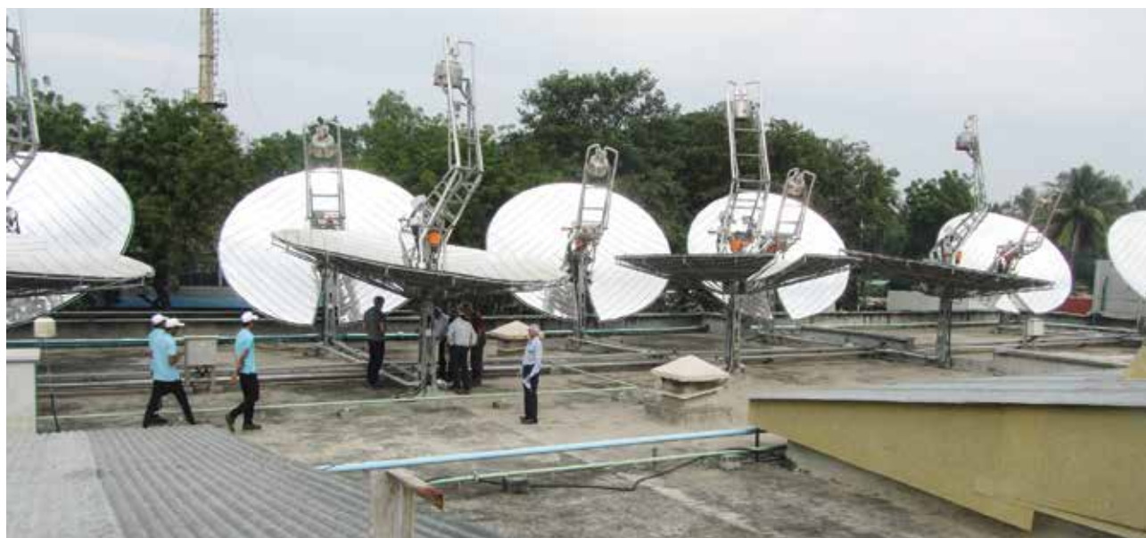
Figure 1: SHIP system at Vidya Dairy for process heating
